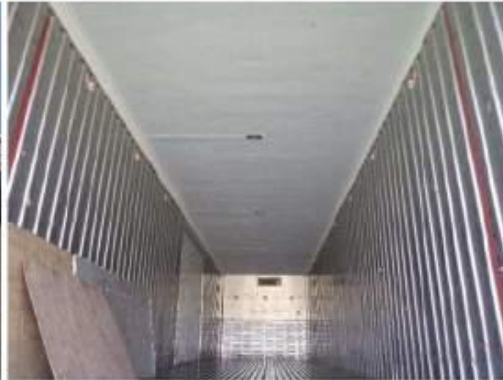
▲ After painting the ceiling
